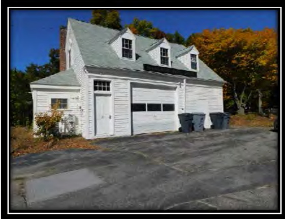
Ayer Road Substation
