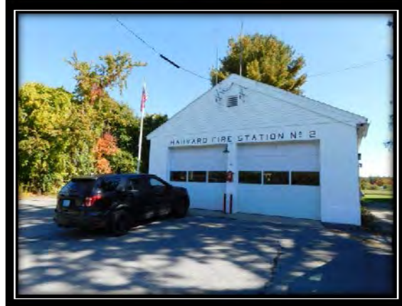
Still River Road Substation
