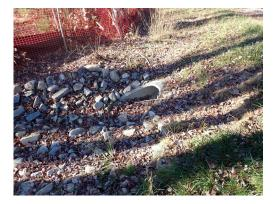
The constructed wetland is acting a sediment basin during construction, however silt in this basin has reached levels that should be addressed to avoid adverse impacts to the wetland resource areas.
