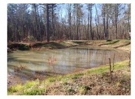
Parabolic Channel (PS8) in front of Building #1 is constantly full of silt. Stabilization of issue with riprap, erosion control barriers and silt sacks have only exacerbated the problem. Proper installation and maintenance of this and all of the Parabolic Channels shall be adhered to.
