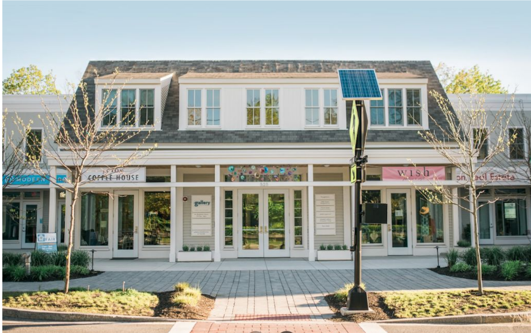
VillageWorks, West Acton, MA Mixed-use Retail / Restaurant / Brewery / Office / Event Space (35,000 sf)
