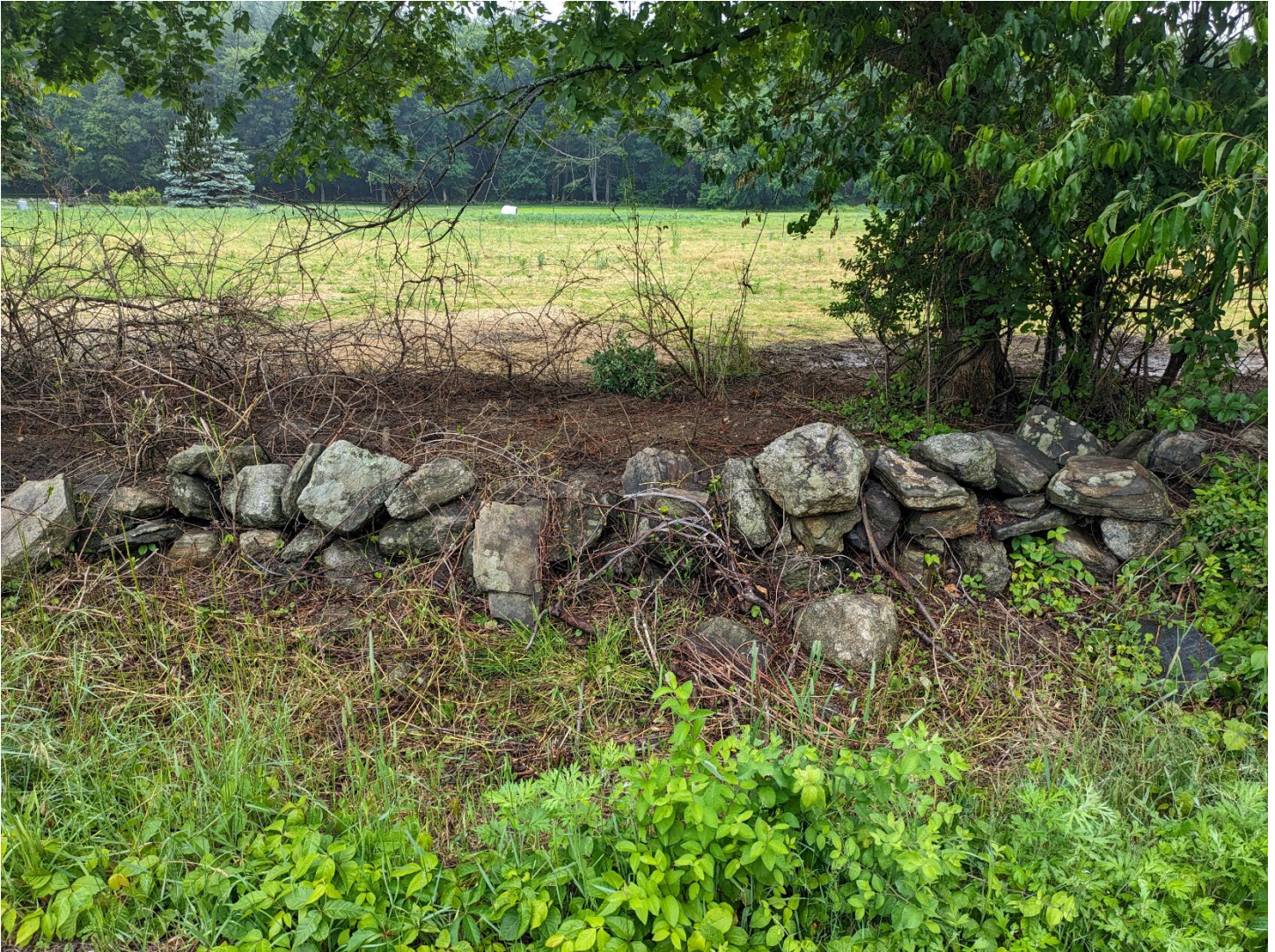
Section of subject wall with invasive vegetation cleared.
