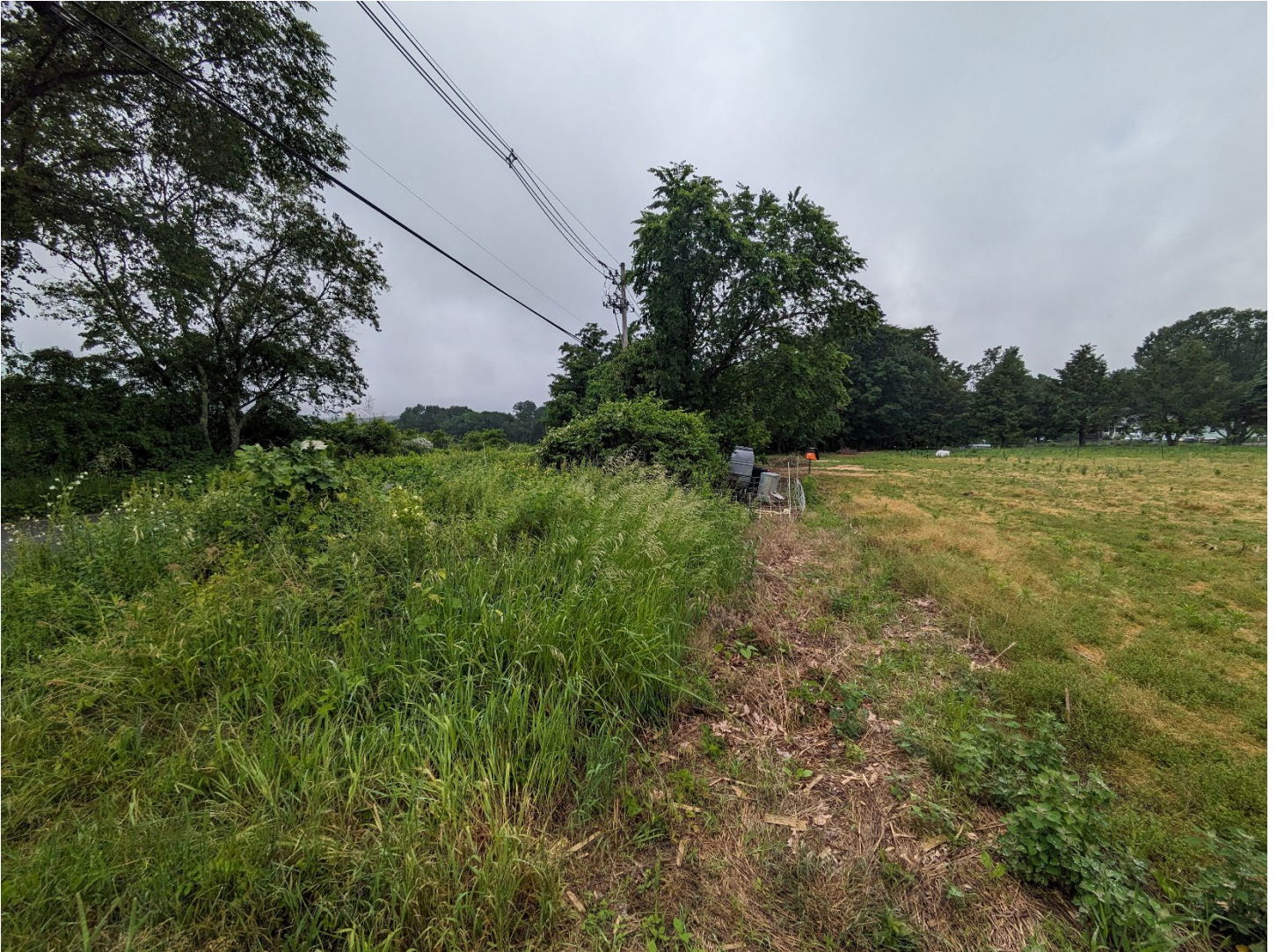
View of subject wall as seen from the property facing Littleton Country Road, looking to the west.
