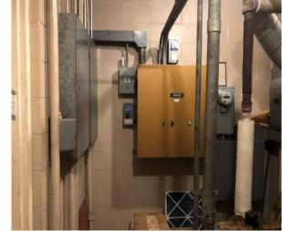
3. The building is equipped with a single double-tub electrical panel which serves all loads/equipment (except the Plymovent system). The panelboard appears to be original to the building's construction and currently does not have space for the installation of additional circuit breakers (panel is full). It
