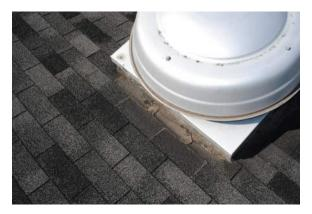
Waves in the shingles were observed one the north side. It appears that the roof deck may have begun to delaminate. Further investigation is required.
