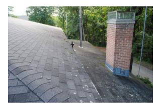
Step flashing at roof to wall locations appears to be in good condition, however, the face is not sealed in a reglet and water can readily infiltrate the roof and building.
