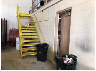
The 7-1/2" raised floor elevation from the break room to the garage floor does not meet accessibility requirements and it also creates a tripping hazard.
