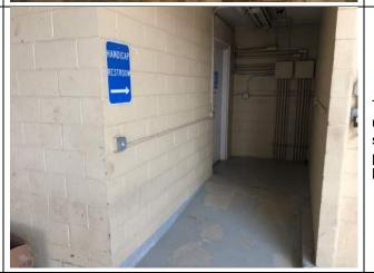
The existing ramp leading to the unisex bathroom exceeds the slope requirements of 1/12 pitch. It also lack handrails on both sides.
