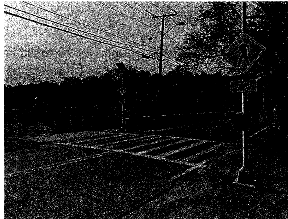
Figure 1: Crosswalk paint markings are faded and illegible.
