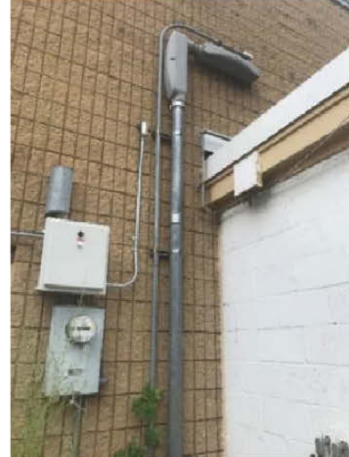
Service Entrance – Exterior of Six Bay Vehicle Storage Garage
