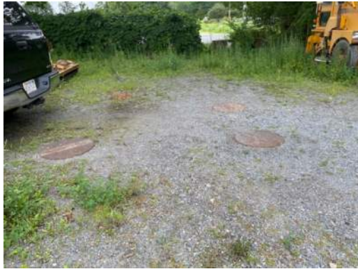
Exterior Tight Tank Manhole Cover located at the Mechanic's Service Garage
