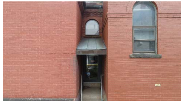
Photo 13: View of the standing seam metal roof area.
