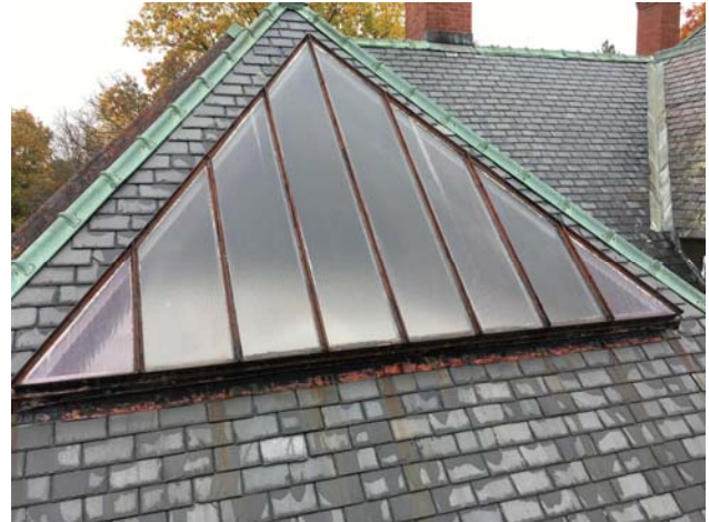
Photo 38: Overview of one of the skylight assemblies.
