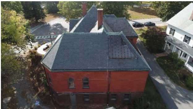
Photo 11: Overview of the slate roof areas at the Old Library.
