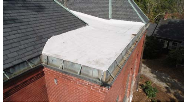
Photo 12: View of the white fluid-applied low-sloped roof area.
