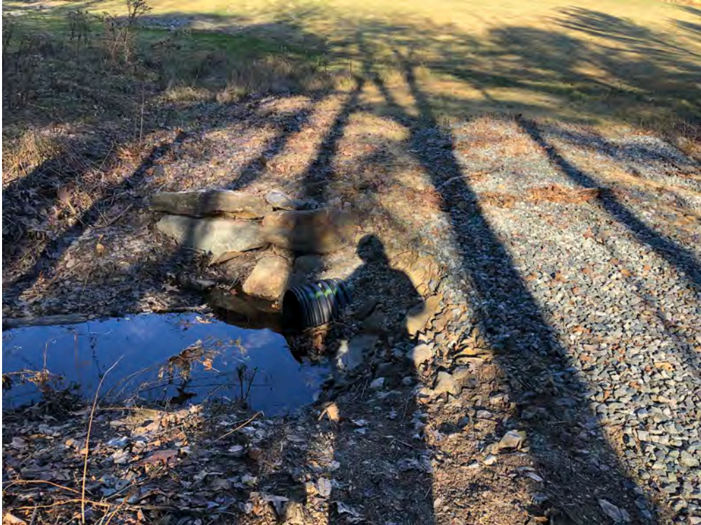
[Site Photo 4 – Facing north at 18” culvert inlet from reconstructed gravel crossing]
