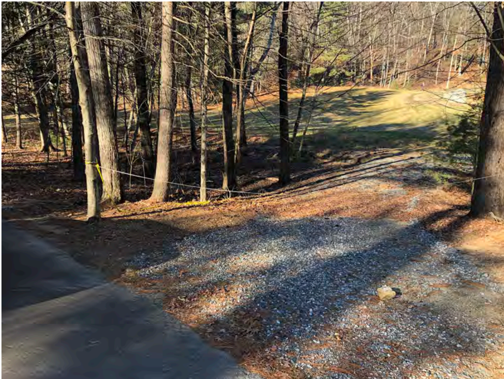
[Site Photo 2 – Facing north at reconstructed gravel crossing from emergency turnaround]
