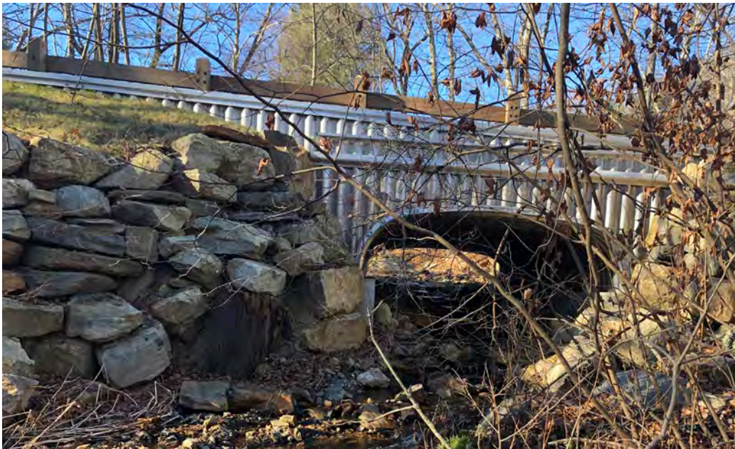
[Site Photo 8 – Stream crossing facing west from easterly side of stream]
