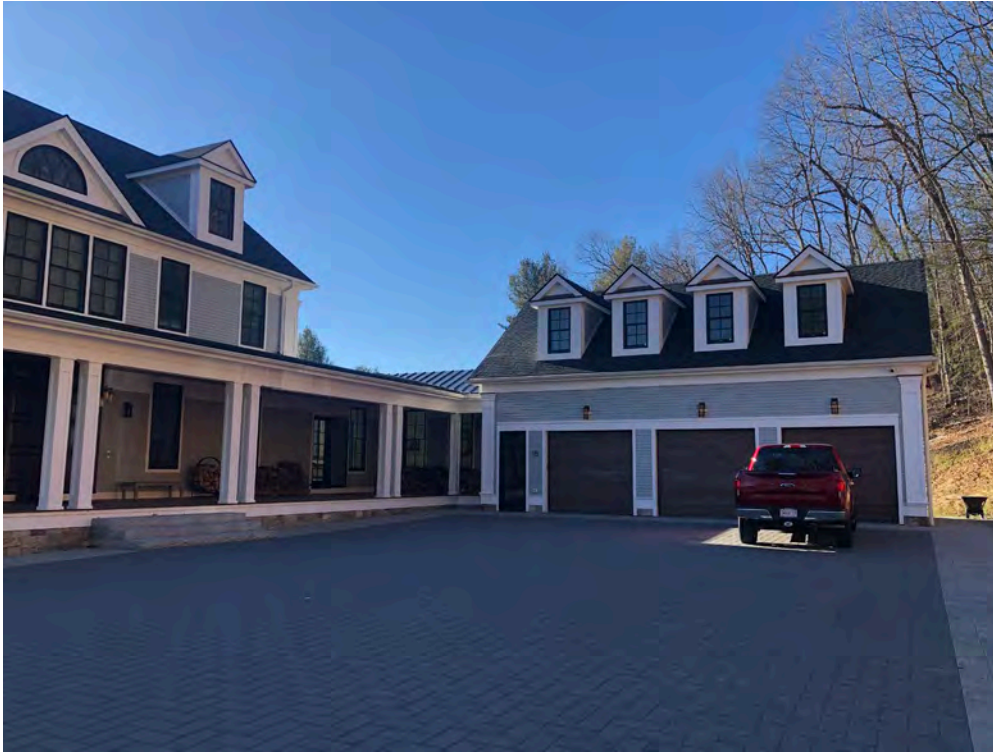
[Site Photo 1 – Facing southwest toward dwelling/garage from driveway]
