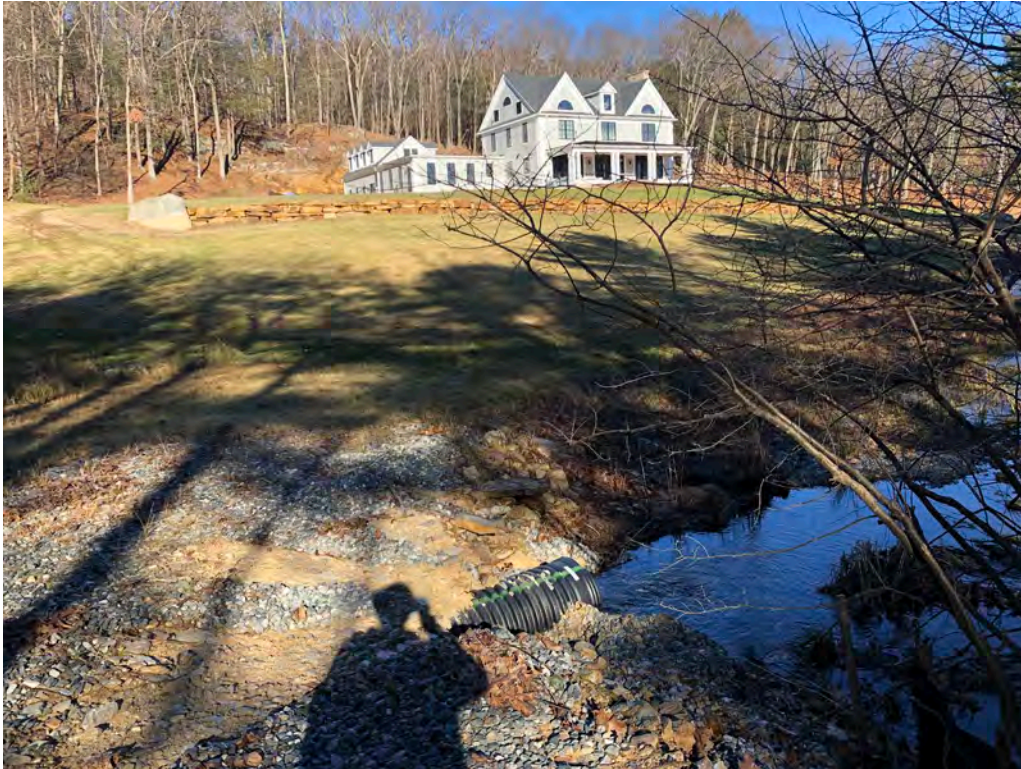
[Site Photo 3 – Facing north at 18” culvert outlet from reconstructed gravel crossing]
