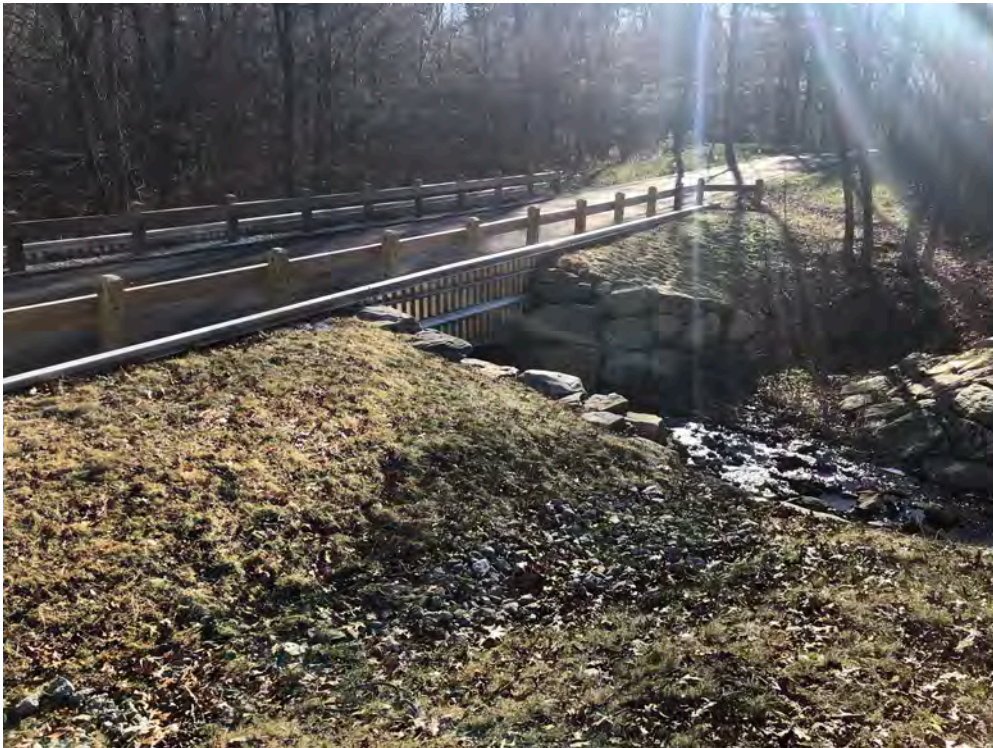
[Site Photo 10 – Stream crossing facing southwest from northerly side of crossing]
