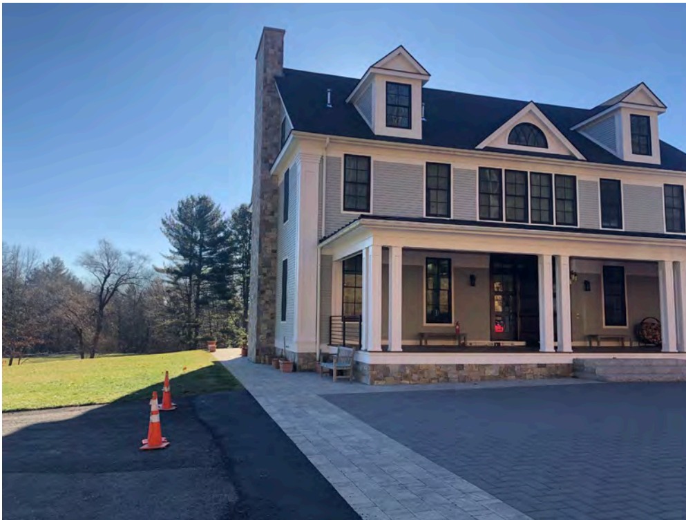
[Site Photo 2 – Facing south toward dwelling from driveway]
