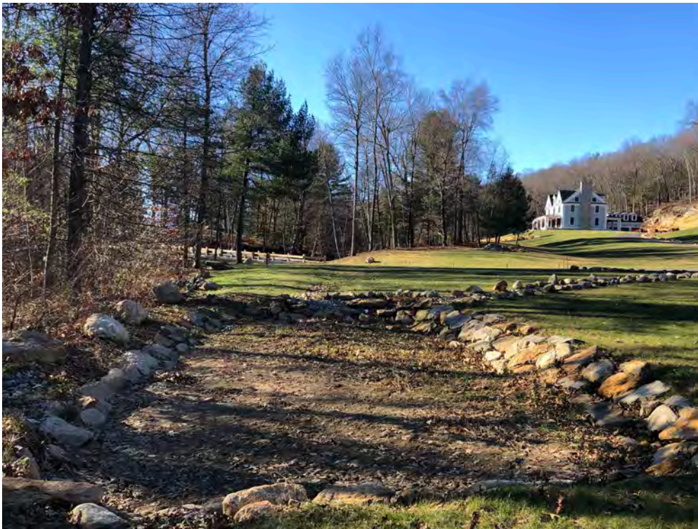
[Site Photo 5 – Facing south at infiltration basin (foreground), stream crossing (background)]
