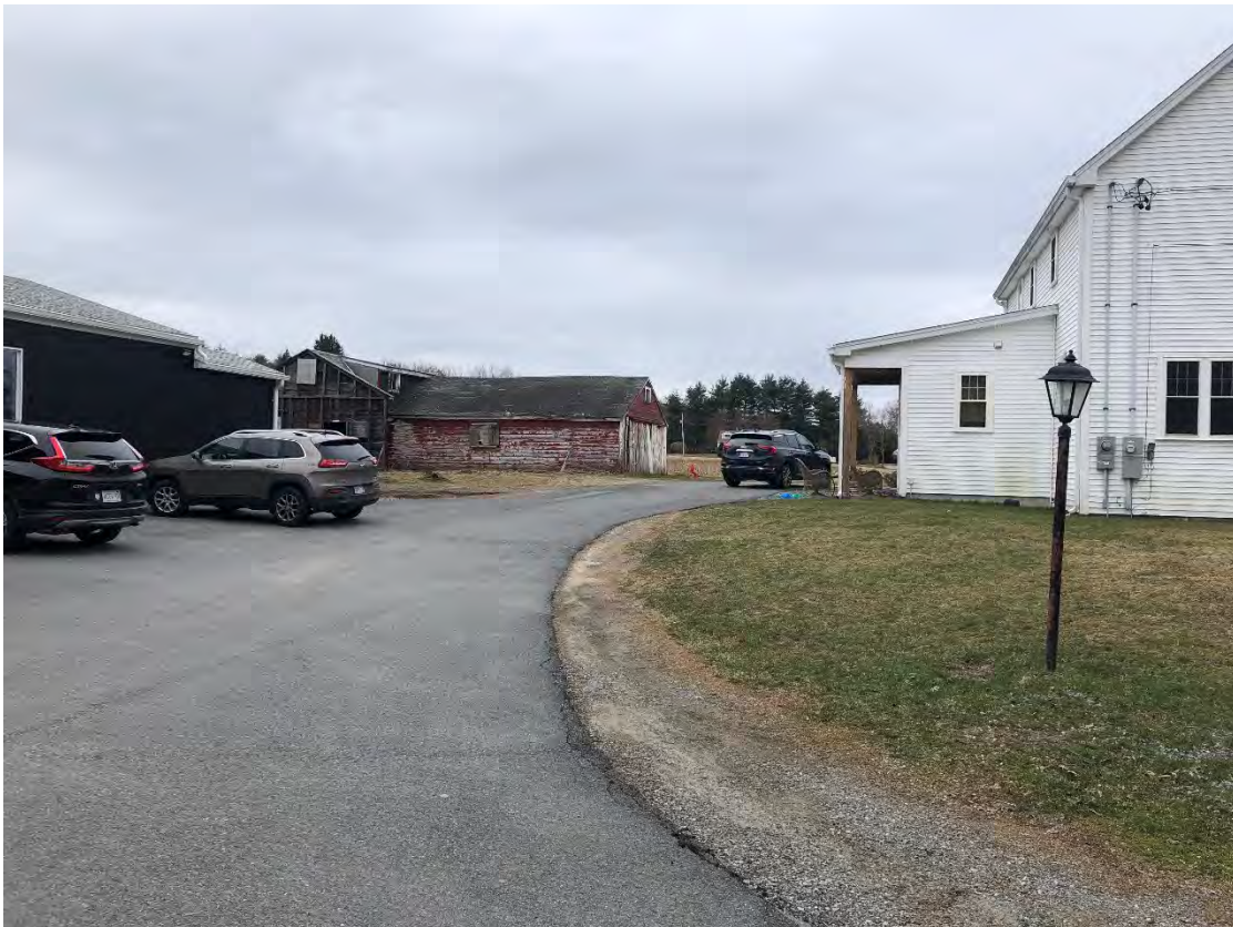
Photo 2: Facing south from northerly most driveway. "The Barn" (left), garage (center) & dwelling (right).
