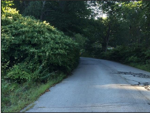
Roadway sight distance and safety issues
