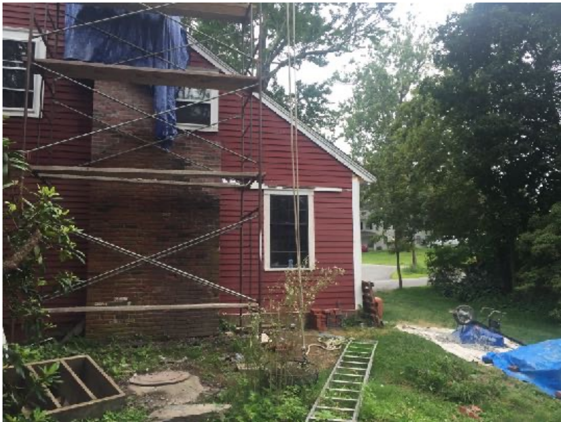
View of site from backyard showing work partially completed. Contrast between old and new brick can be seen.
