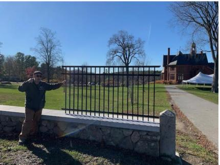
The proposed fence would include a 2-foot stone wall with a 4-foot metal railing. The metal is a powder coated aluminum in black — matching the grill over the window on the building.
