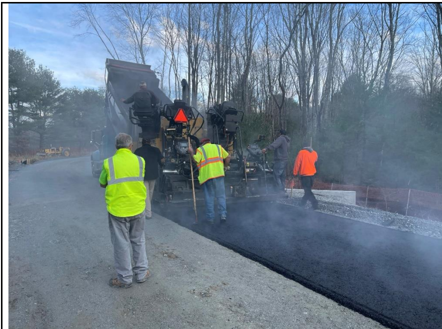
Contractor used a larger paver to pave the Pine Banks road.
