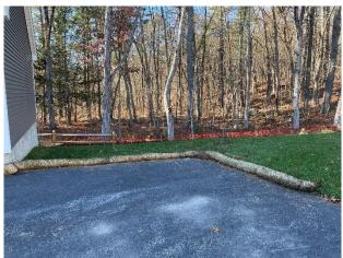
3. Nitsch observed that the material for the septic system near Unit #8 has eroded and flowed off property. Nitsch recommends that the Contractor stabilize the material and remove and dispose of properly, the material that flowed off site into the abutting property (Phase 2).
