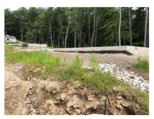
5. The Contractor shall provide a permanent solution for the low point at the roadway intersection with Stow Road so that water flows toward the wetland. The Conservation Agent agreed that a swale toward the wetland was an appropriate temporary solution. The Contractor shall provide a detail with spot grades that indicate how the permanent condition will be constructed.
