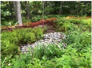
4. The Contractor shall re-establish any silted bio-retention systems and protect completed bio-retention systems with erosion control measures if the contributing drainage areas to the bio-retention systems are not stable and vegetated. Silt and sediment in the bio-retention systems shall be removed and disposed of properly and not reused in the bio-retention systems.
