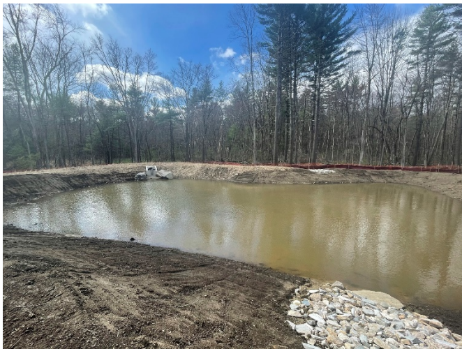
Sediment is visible in the constructed wetland.
