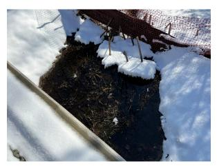
8. Contractor had built a bump or asphalt curb along the access road to the houses 5 and 7 to prevent stormwater and sediment from running in to the driveway. Contractor to provide a sketch approved by the design engineer, and a written statement to show how this solution is adequate in the interim construction condition and in the final condition. Also, it appears that the installed ramp had eroded in some area.
