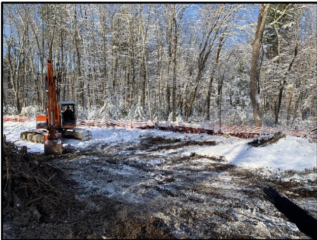
Figure 3 – cleared trees leave behind a tremendous amount of sediment that is susceptible to being washed into the stream.
