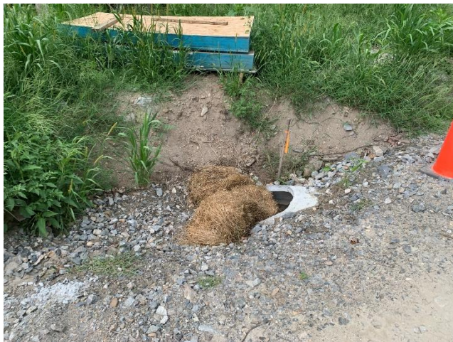
Picture 1 – Hay bale was placed at inlet.
