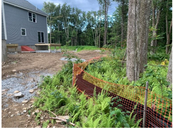
Picture 3 – Fence is in good condition with wattles intact.
