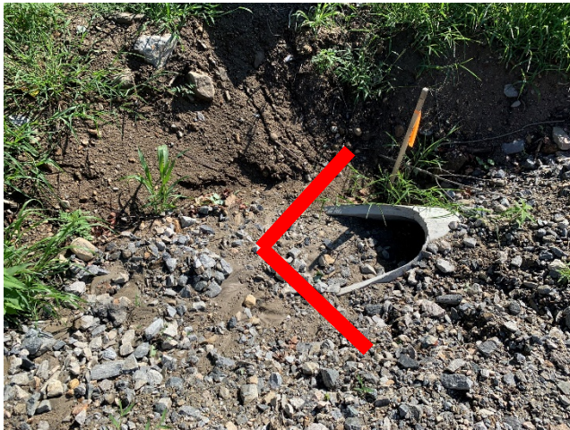
Picture 1 – Sediment buildup around flared end inlet which drains to constructed wetland.
