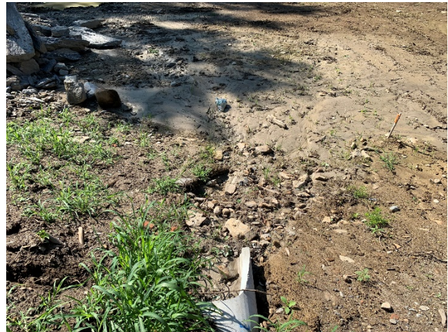
Picture 2 – Sediment entering constructed wetland from upstream inlets.
