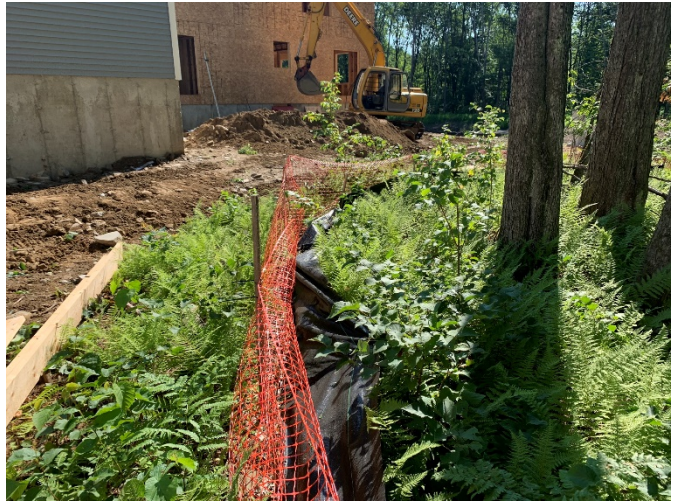
Picture 4 – Erosion control barrier has been damaged.
