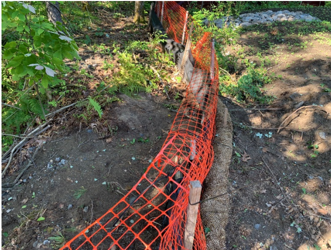
Picture 3 – Some sediment is shown crossing over erosion control barrier offsite. It is recommended hay wattles be replaced on both sides of fence.
