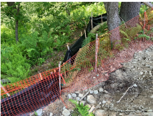
Picture 3: Erosion Control
