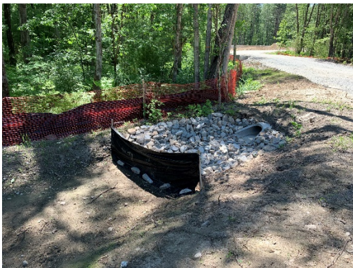
Picture 1: Bioretention Cell
