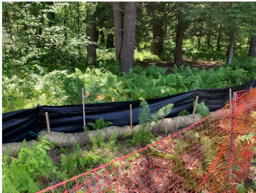
Picture 4: Erosion Control
