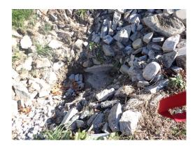
A major cause of siltation with the Parabolic Channels and Constructed wetland is the uncontrolled runoff from the upper portion of the site. A plan to properly control stormwater runoff shall be submitted to the Commission for their review.
