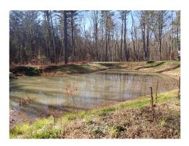
Parabolic Channel (PS8) in front of Building #1 is constantly full of silt. Stabilization of issue with riprap, erosion control barriers and silt sacks have only exacerbated the problem. Proper installation and maintenance of this and all of the Parabolic Channels shall be adhered to.
