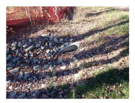
The constructed wetland is acting a sediment basin during construction, however silt in this basin has reached levels that should be addressed to avoid adverse impacts to the wetland resource areas.
