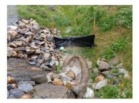
Parabolic Channel 7 (PS7) was designed to be a series of step pools along the main road of the development. As constructed this channel is one long channel that has been stabilized sporadically similar to PS8. Proper installation and maintenance of this and all of the Parabolic Channels shall be adhered to.
