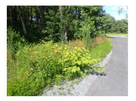
The lower Bio-Retention Cell is receiving silt during rain events. Areas in which stormwater is flowing shall be stabilized to reduce silt from entering this cell.
